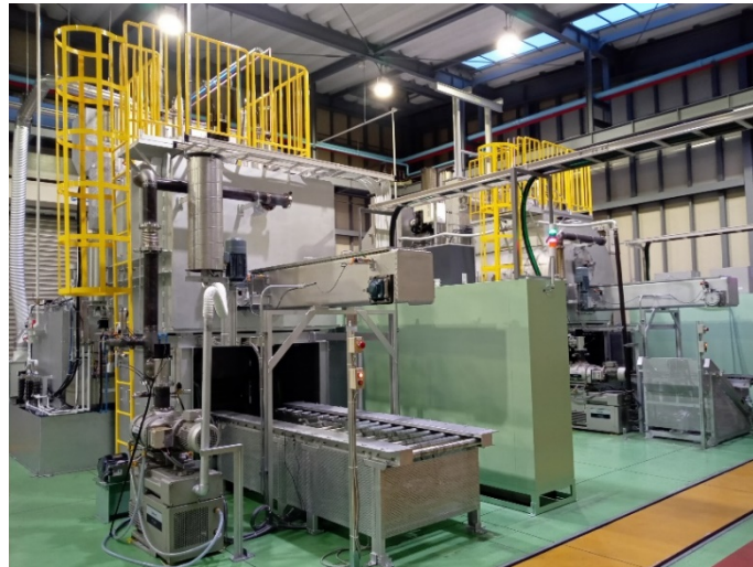
The Z-TKM installed at the Hamamatsu Plant
