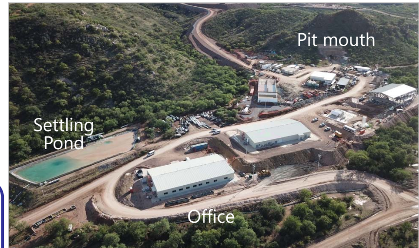
Los Gatos Project-Status of Construction
