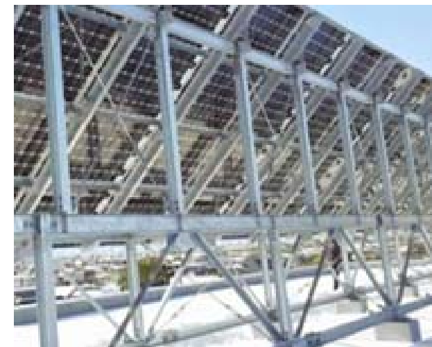
Example of a next-generation panel (power generated from both sides of the panel) 15
