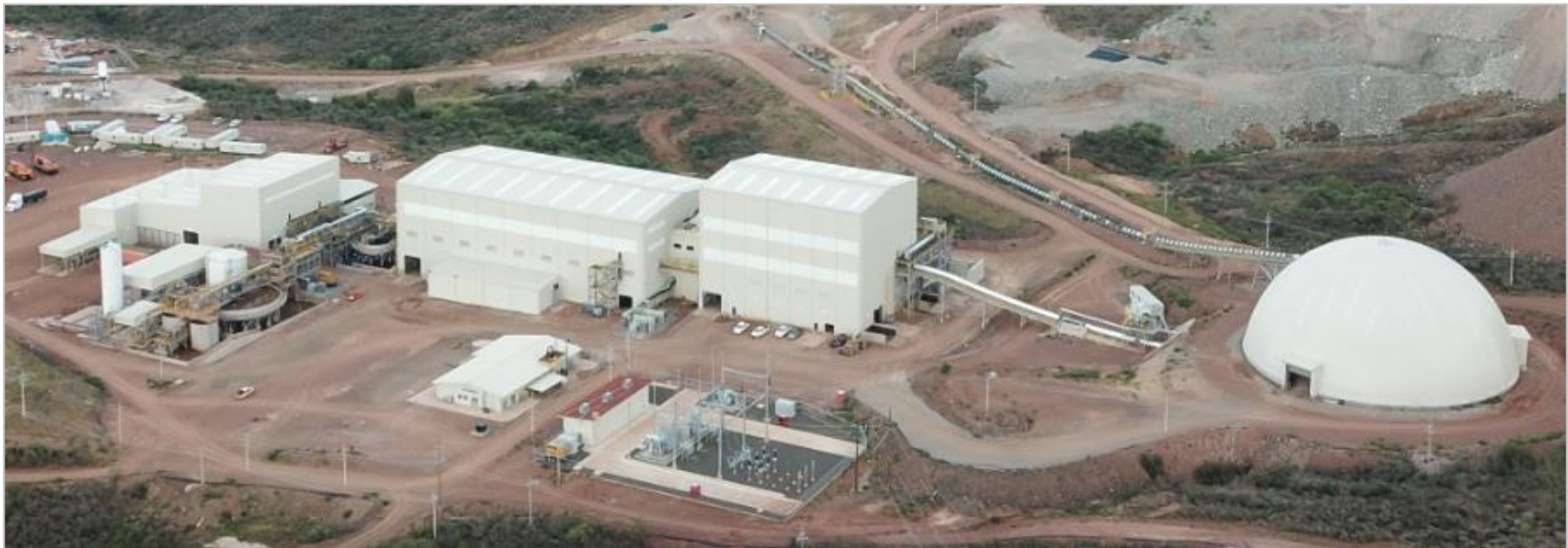
Overview of Process Plant and Stockpile Dome
