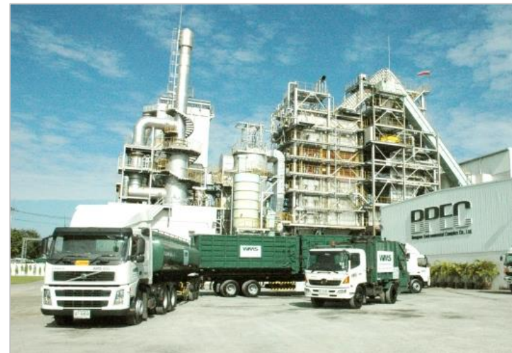
Incineration Plant in Thailand
