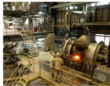
PGM recovery plant
