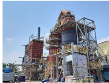
The incinerator is under construction in Indonesia.
