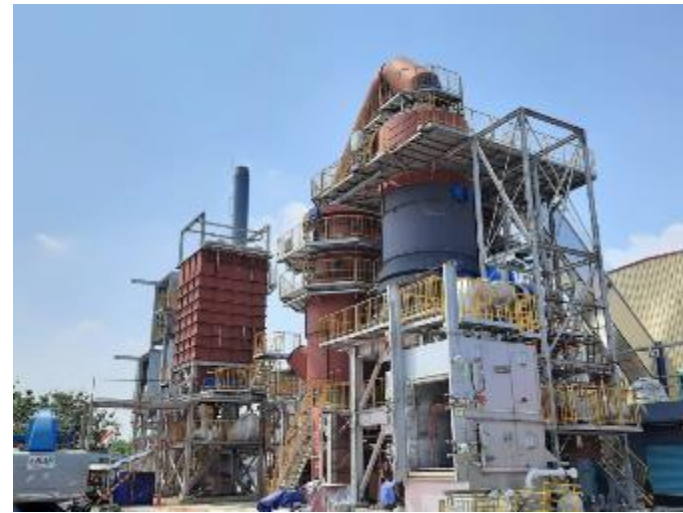
The incinerator is under construction in Indonesia.
