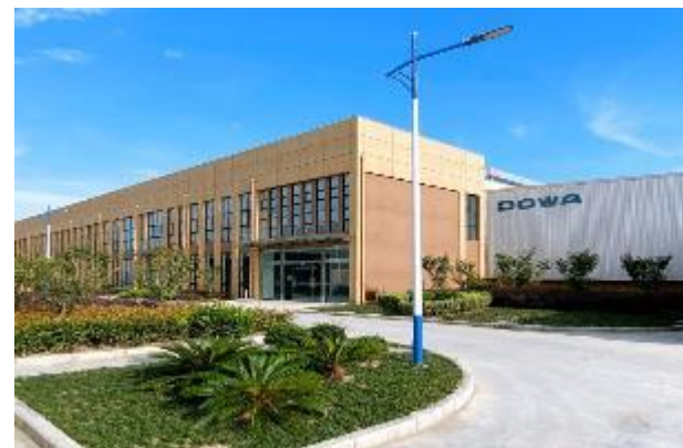
New factory in China (DOWA METALTECH (NANTONG))
