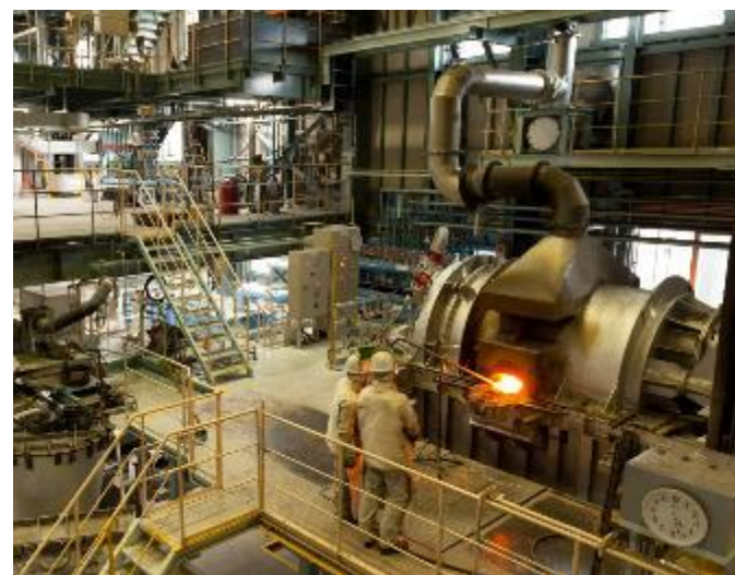
PGM recovery plant
