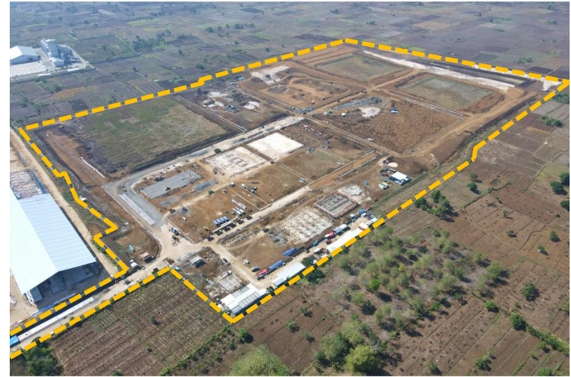
Second landfill site (under construction)
