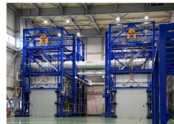
Heat treatment facility in Akita
