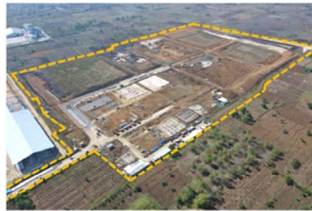
Second landfill site (under construction)
