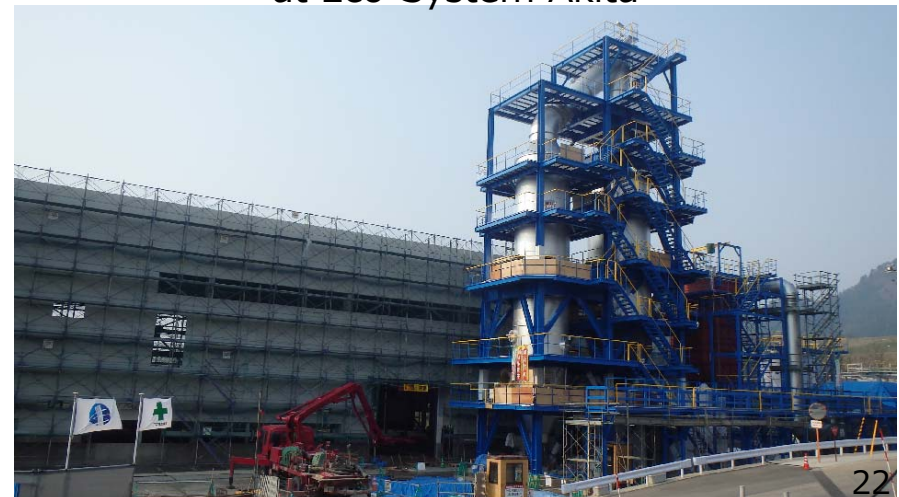
Construction of PCB waste treatment facility at Eco-System Akita
