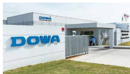
Our zinc processing plant in Thailand
