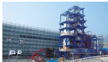
Low-contaminated PCB treatment plant under construction in Akita
