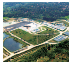
Controlled landfill in Indonesia
