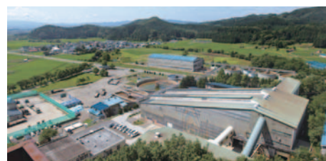
Contaminated soil remediation facility, Eco-System Hanaoka Co., Ltd.
