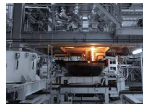
Waste melting and recycling facility
