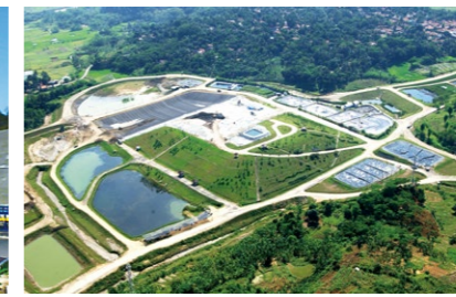
2009: Began waste treatment in Southeast Asia
