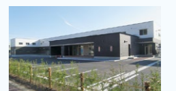
Dormitories for single employees in Kosaka, Akita Prefecture that were renewed in 2018
