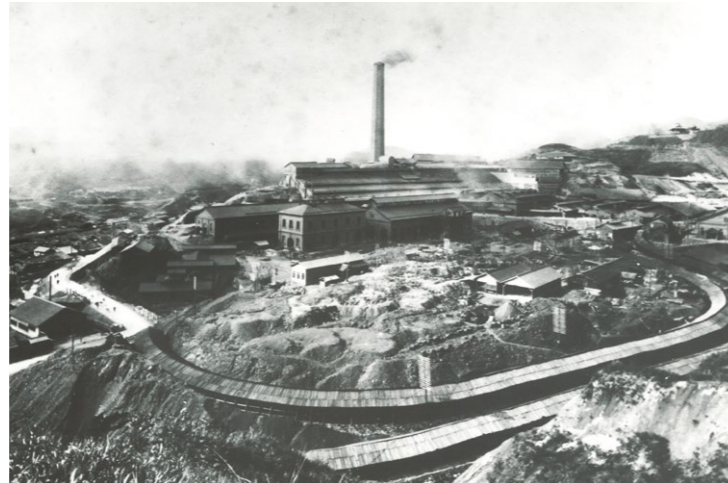
1907: Roaster at Kosaka mine (currently Kosaka Smelting & Refining Co., Ltd.)
