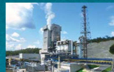
Kosaka Smelting & Refining after its conversion to recycling and smelting operations
