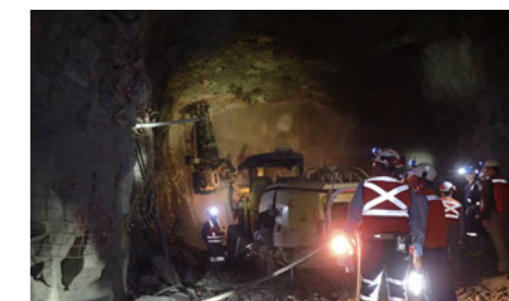
Mine construction at the Los Gatos Silver, Zinc, and Lead Project
