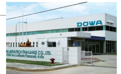
Precious metals electroplating plant in Thailand
