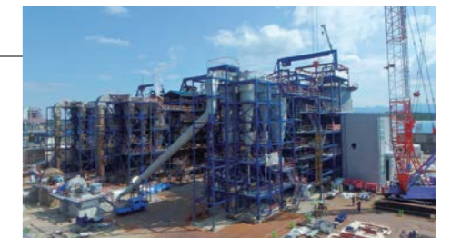
Building and renewing roasting furnaces underway at Akita Zinc
