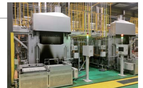
Heat treatment processing facilities
