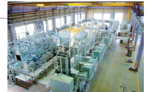
Heat treatment furnace manufacturing plant
