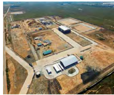
Controlled landfill facility for waste, constructed in Myanmar
