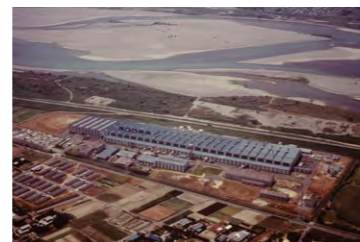
Around 1980: Toyooka Plant (currently DOWA Metal Co., Ltd.)
