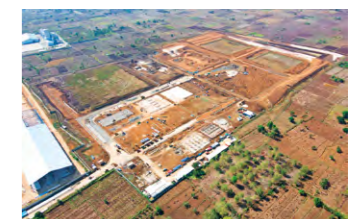
Second base in Indonesia (under construction)
